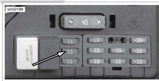
Figure 7-11. Fuel Pump Fuse
