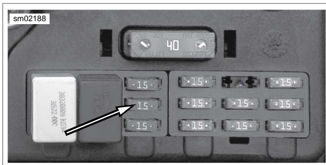
Figure 4-33. Fuel Pump Fuse
