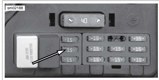
Figure 4-13. Fuel Pump Fuse
