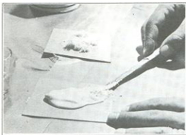
Figure 2J-2. Mixing Gel Coat and Glass Fibers
