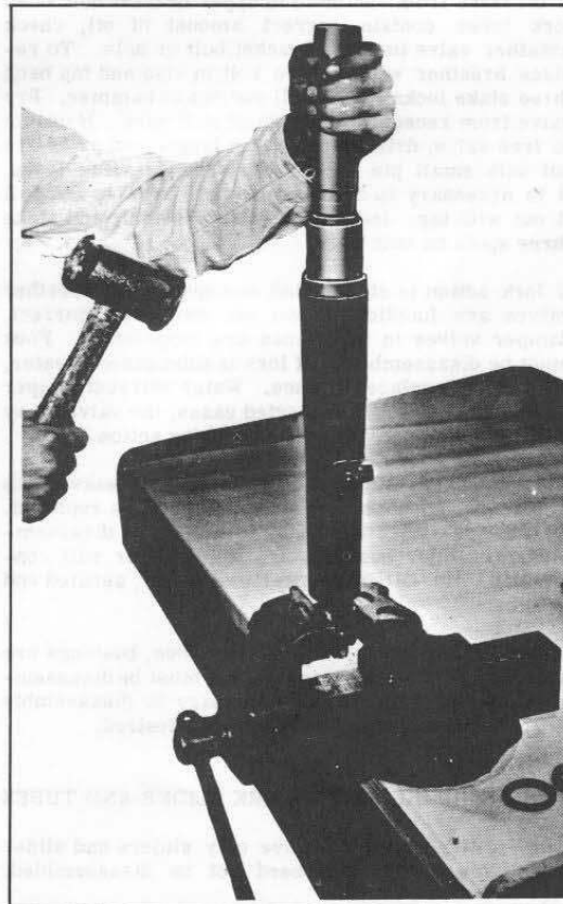
Figure 2F-7. Driving in Fork Slider Bushing
