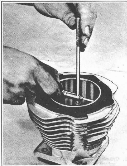
Figure 3C-4. Measuring Cylinder Bore
